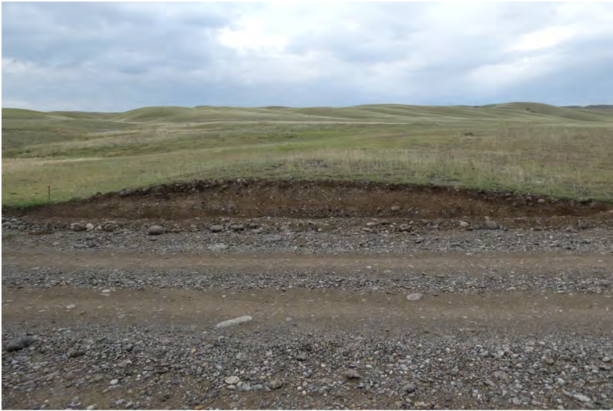
Fig 6. Exposed section of Kurgan no. 1 at site GS011 damaged by road construction
