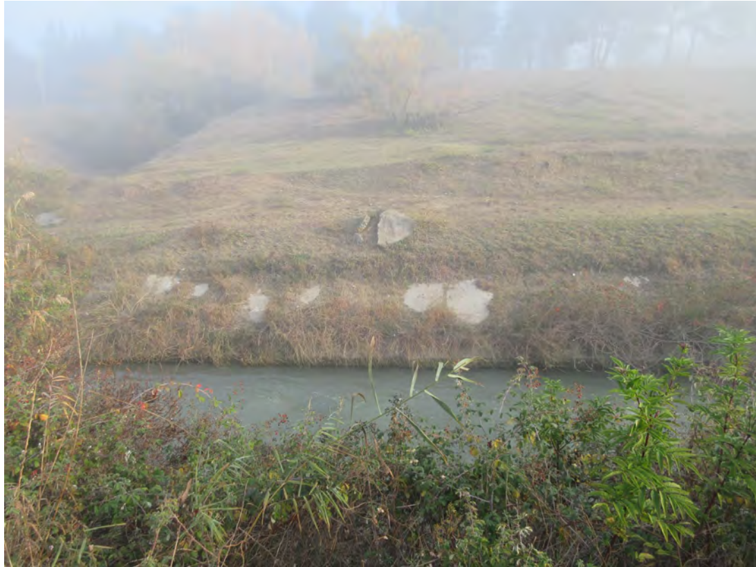
Fig. 8. View of the main Mariini Canal (site GS045) close to its southernmost point, from W, with visible Soviet modifications (above); view of the possible abandoned branch of the same canal from NE (below)
