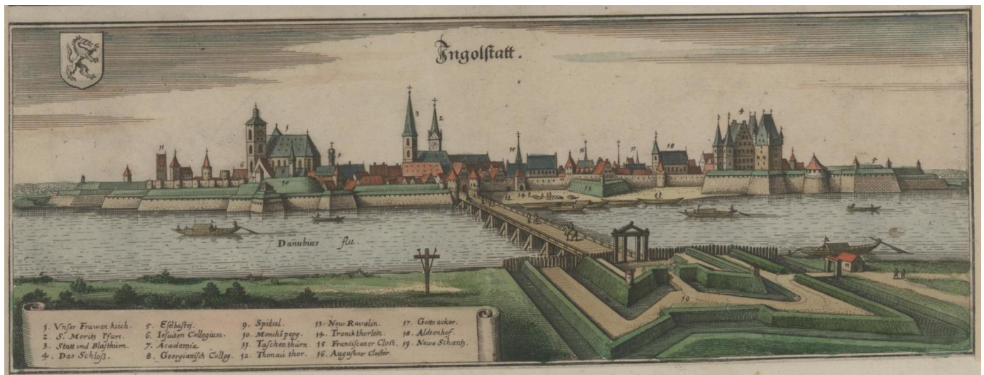
The Bavarian fortress at Ingolstadt seen from the south: 16th century waterworks and fortifications with minor 17th century additions (Matthäus Merian, 1644) (SLUB Dresden / Deutsche Fotothek)
