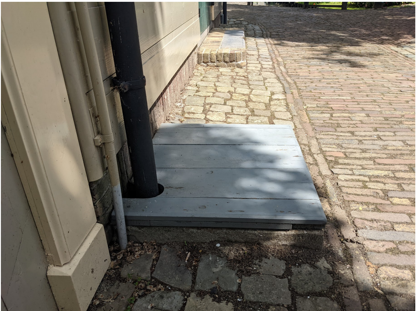
A street cistern in Amsterdam. Photo: author
